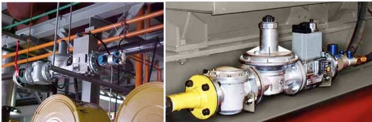
Typical GTI Bi-Fuel Gas Train Mounting Options: “Trapeze” Method (left), and “Bottom” Method (right)
